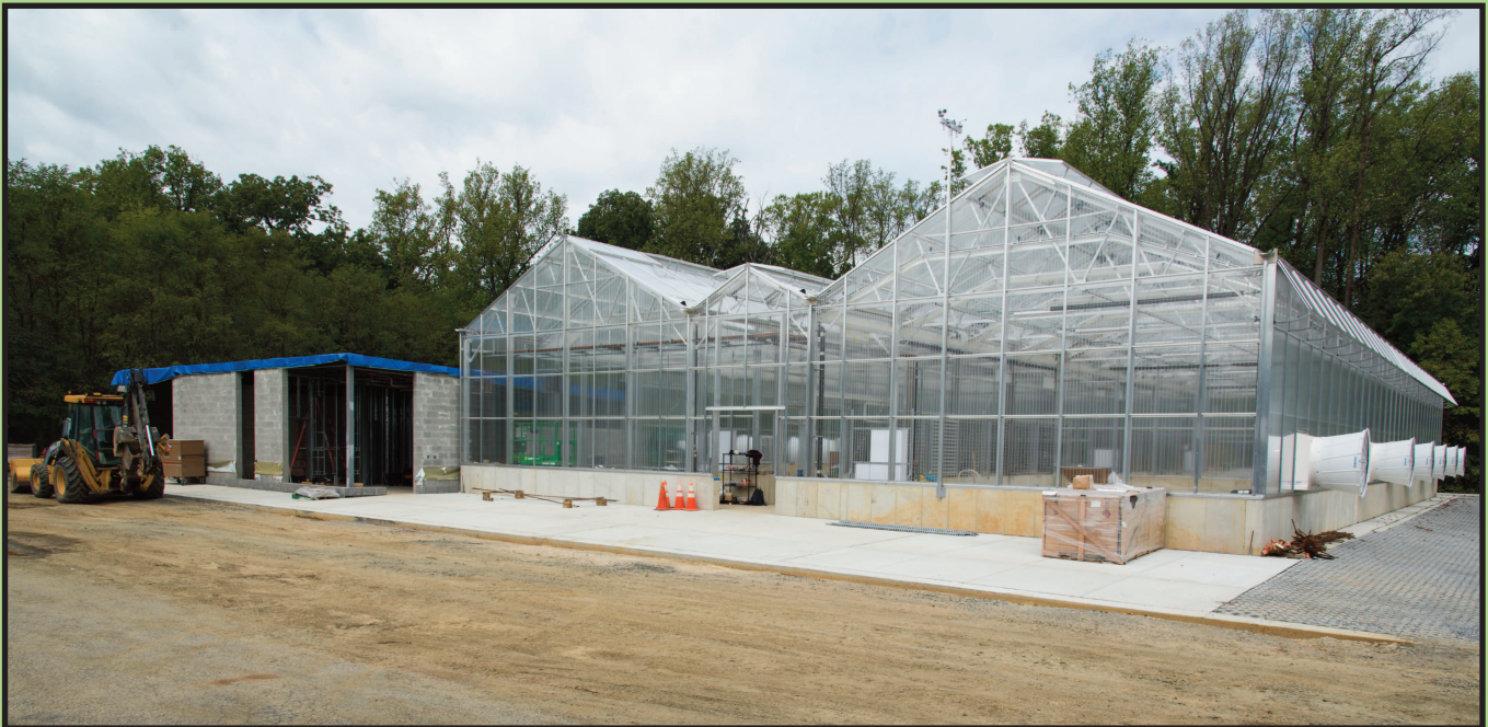
A recent view (20 September 2023) of the new Botany Research Greenhouse range under construction at the Smithsonian Museum Support Center (MSC) in Suitland, Maryland. The greenhouse structure is complete with ongoing work on utilities and the headhouse. The expected completion date is January 2024. (photo by K. Wurdack)
