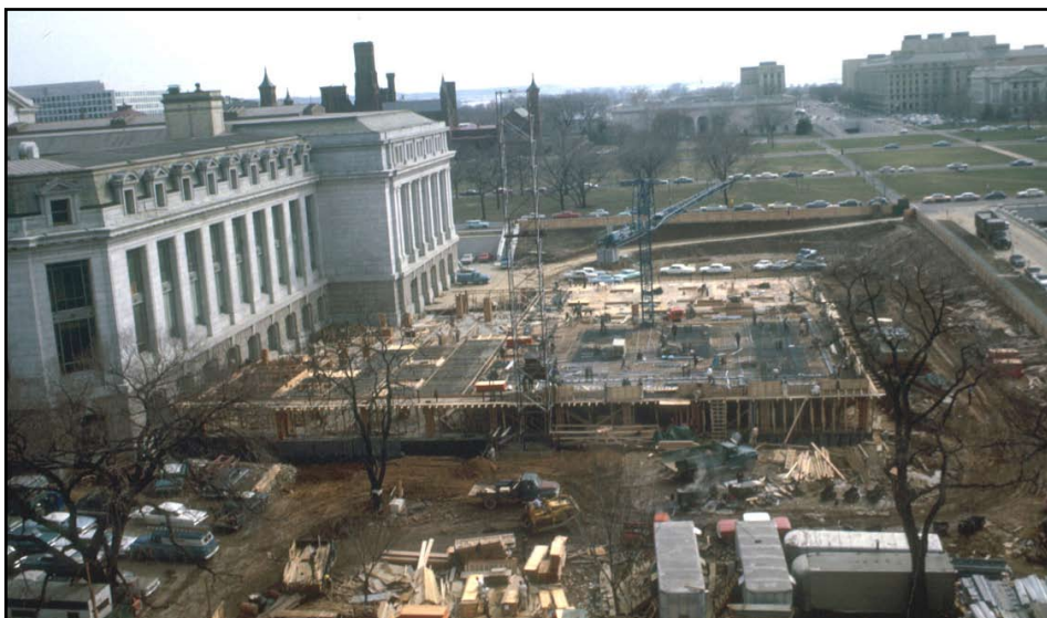
Construction of the West Wing of the National Museum of Natural History (future home of the US National Herbarium) in their early 1960s.
