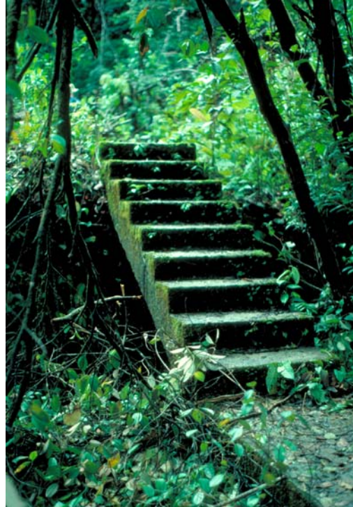
Plate 7: One of the cement steps built during British rule along the path to Johnson's View.
